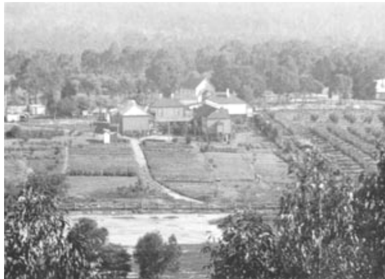
Figure 4 – The Salvation Army's Bayswater Boys Home at The Basin
